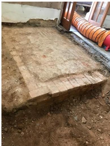
Last week I talked a bit about the 'Pool family' vault and this picture shows it a little closer-up. The Structural Engineer will be looking at it later in the week so we will then know if it will stand a layer of stone above it, plus people on the floor, without collapsing. The top of the vault is a very shallow arch so it might need strengthening a little but more on that next week.
